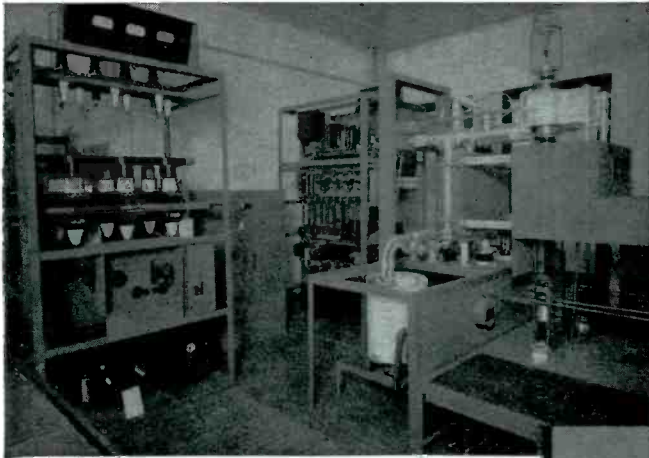
(Above) PROGRESS IN FM BROADCASTING offers an expanding field for Isolantite*—the logical insulation choice for this and other types of radio work. Photo shows the 50KW FM transmitter built by Radio Engineering Laboratories, Inc., for The Evening News Association, Detroit—the third unit of this type to go on the air. Plate lines and other units are supported by Isolantite insulators. Photo at right shows close-up of power amplifier unit.
